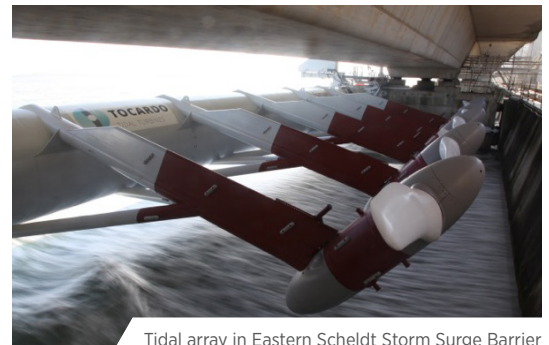
Tidal array in Eastern Scheldt Storm Surge Barrier
