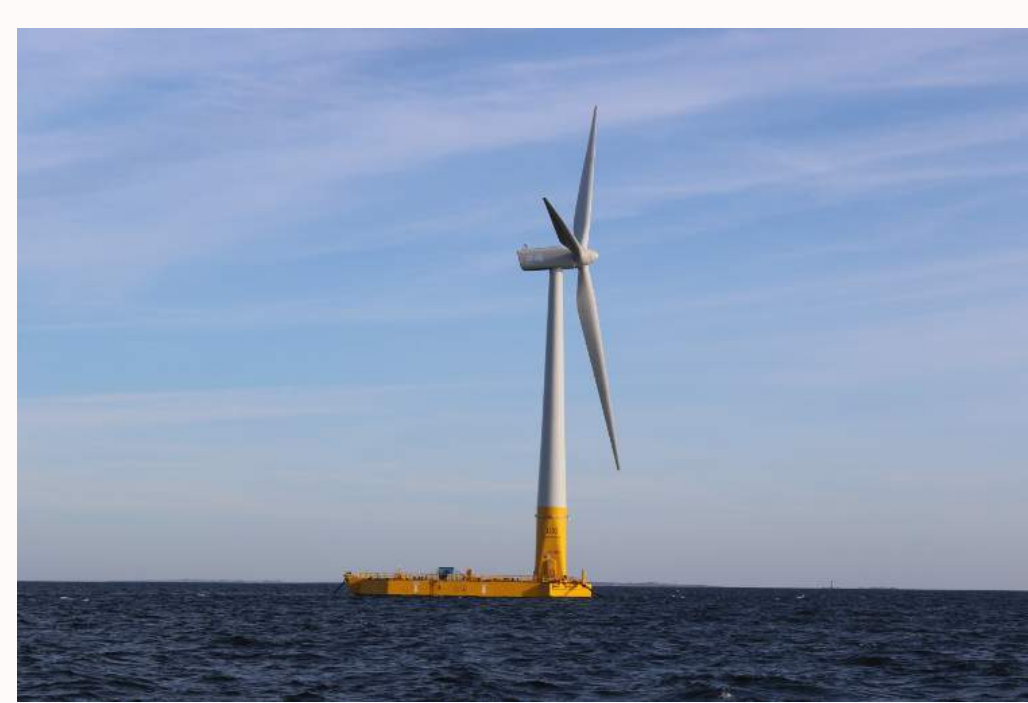
Figure 1: FLOATGEN, the prototype at SEM-REV test site in Le Croisic (France) 4 .
