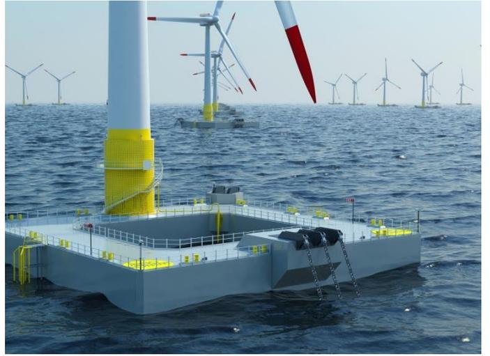
Figure 1. Floatgen FOWT Reinforced Concrete substructure. Courtesy of BW-IDEOL.
