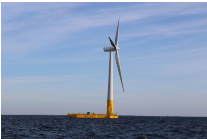
Figure: FLOATGEN, the prototype floating offshore wind turbine, used as a reference in this project.
