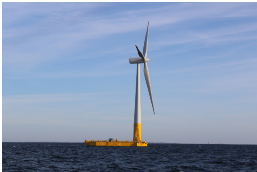
Figure: FLOATGEN, the prototype floating offshore wind turbine, used as a reference in this project. Source: https://sem-rev.ec-nantes.fr/medias/photo/sem-rev-bj-132-bd_1539862739781-jpg?ID_FICHE=196422 Accessed: 2020-09-21
